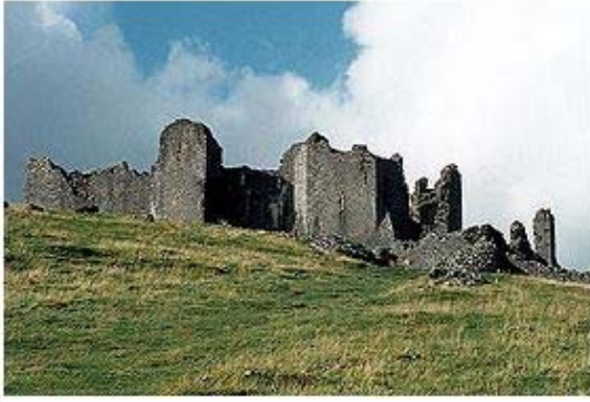
The western front. (photo © Allan Matthews)
